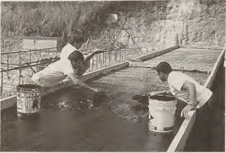
FIGURE 13.7 Beds sealed with bituminous paint. (From Hidroponias Venezolanas, S.A., Caracas, Venezuela. With permission.)
