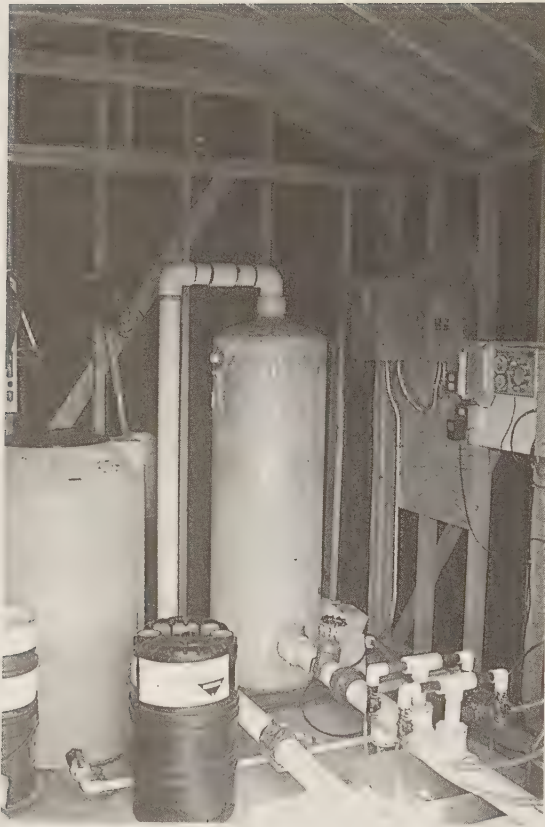
FIGURE 6.56 Injector system with acid tank on left, blending tank in middle, and part of injector system at lower right with irrigation controller above. (From California Watercress, Inc., Fillmore, CA. With permission.)
