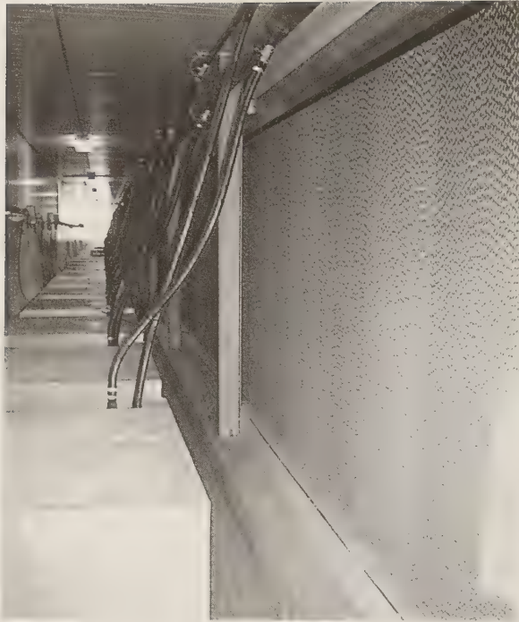
FIGURE 10.32 Positive pressure cooling/heating greenhouse system. (From Eurofresh Farms, Wilcox, AZ. With permission.)
