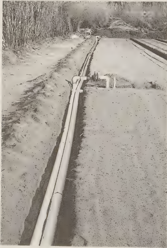
FIGURE 6.49 Irrigation mains at side of field. Four-inch-diameter raw water main and 3-in. nutrient solution main. Note: Risers to solenoid valves of 2-in. submains going across the field. (From California Watercress, Inc., Fillmore, CA. With permission.)
