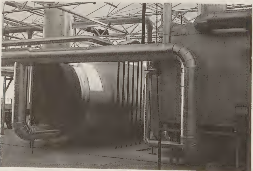
FIGURE 9.7 Carbon dioxide recovery unit attached to central boiler.
