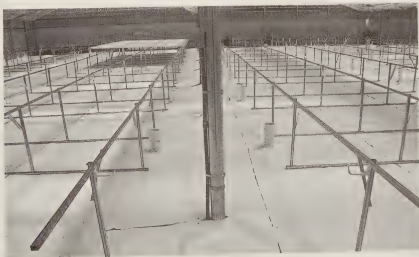
FIGURE 6.4 Benching system constructed for support of the NFT channels. Note: The channels placed on the bench in the back. Also, note that the benches are sloping toward the greenhouse side-wall posts and there are 3-in. PVC drain pipe risers for the catchment trench to drain to for return to the nutrient cistern. (From American Hydroponics, Arcata, CA. With permission.)
