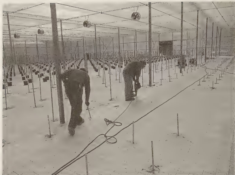
FIGURE 12.36 Placing base conduit support in soil.
