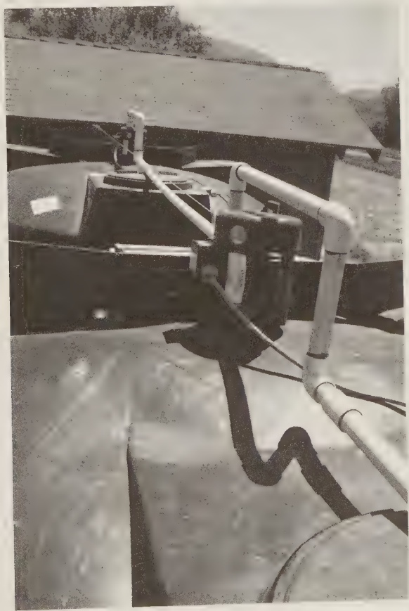
FIGURE 3.7 Stock tanks (2,300 gal) A and B with circulation pumps. (From California Watercress, Inc., Fillmore, CA. With permission.)
