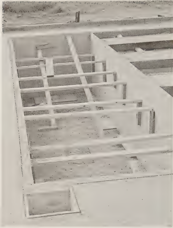
FIGURE 7.7 Nutrient tank construction.
