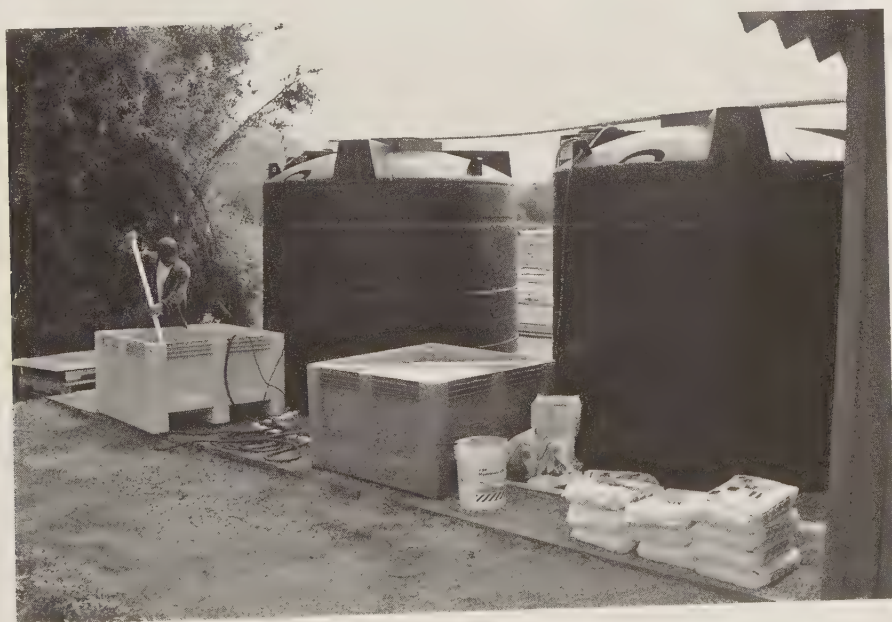
FIGURE 3.9 Image of 2,300-gal stock tanks with injector shed. (From California Watercress, Inc., Fillmore, CA. With permission.)
