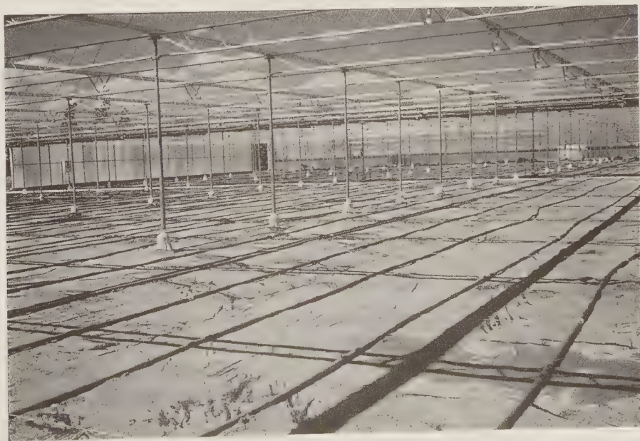
FIGURE 8.3 The laying of a polyethylene liner and drain pipes.
